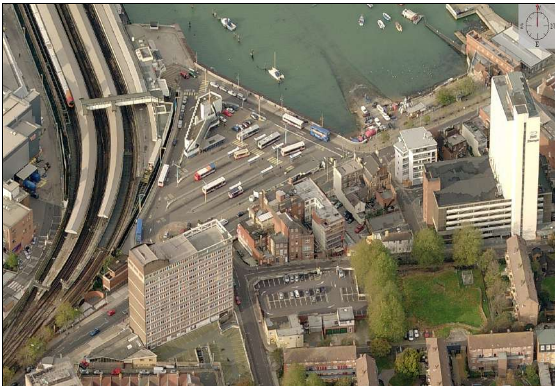
3. Oblique view of Hard from east. Eastern part of 'Sub Area A' including Brunel House and Car park to rear, and Havant Street Car park clearly visible.
