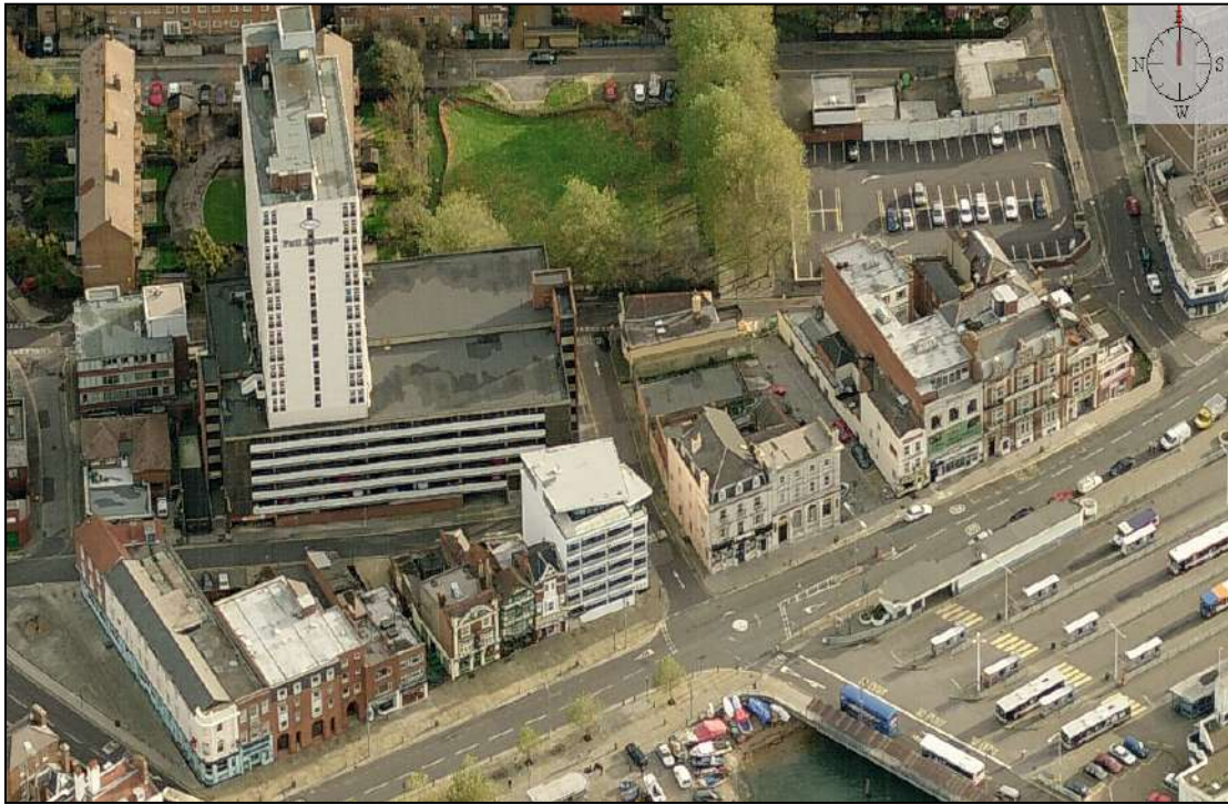
2. Oblique view of 'Sub Area B' The Hard from the west – Europa House Pall Filtration building and multi storey car park clearly visible.
