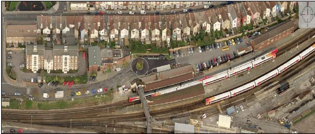
3. Oblique view of 'sub-area C' Fratton from south. The Station car park (top right) and modern block of flats (centre left) are clearly visible
