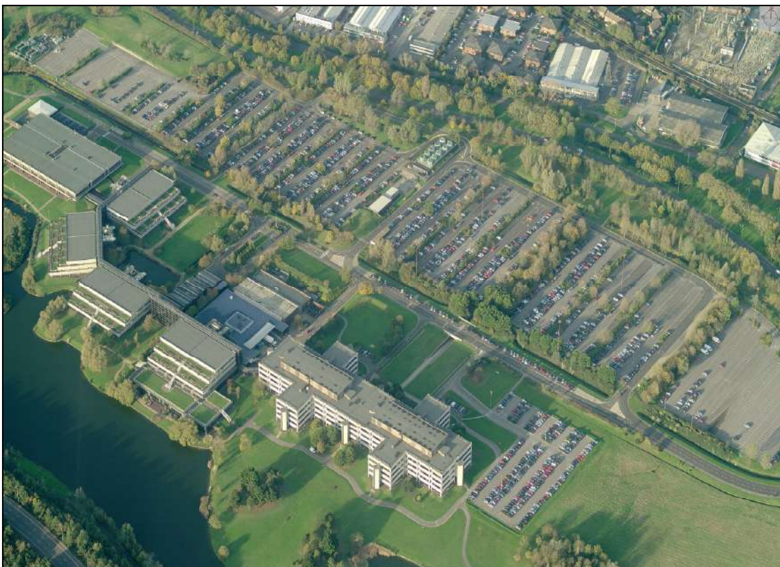
3. Oblique view from the south of sub area B - IBM site
