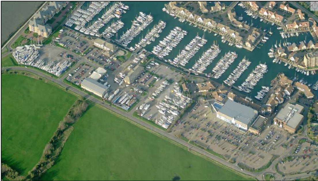
1. Oblique view of 'sub-area A' Port Solent southern part of Port Solent from the south
