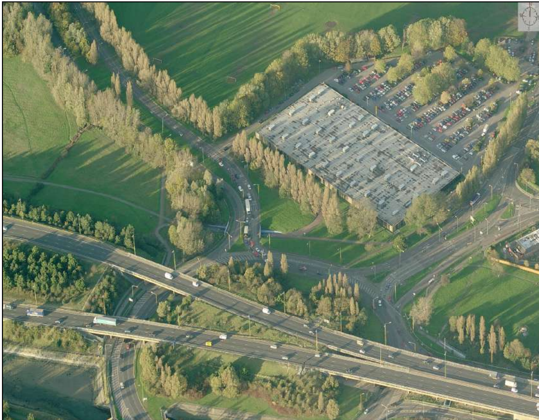
4. Oblique view from the south of sub area B former IBM offices junction of Western Road/Northern Road Cosham.
