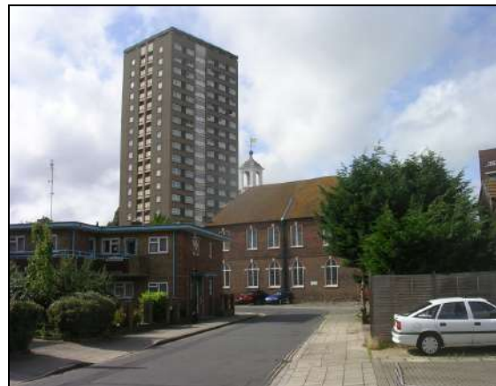
4. View from south east (Britain Street)
