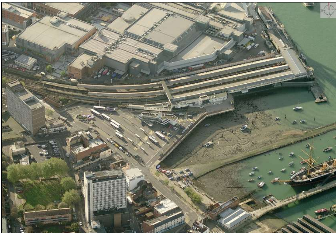
1. Oblique aerial view of entire Hard 'Area of Opportunity' from the north.
