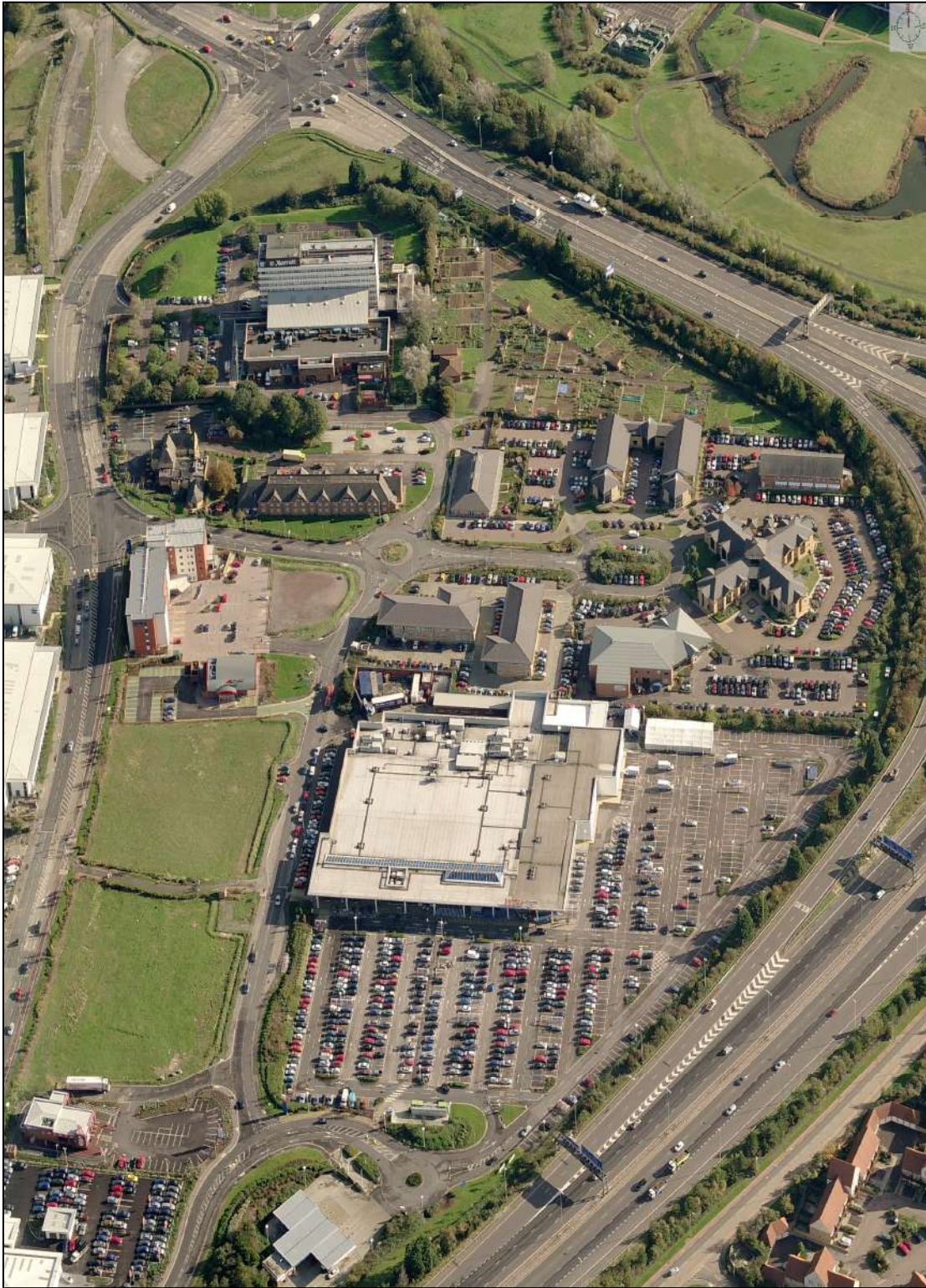
1. Oblique view from west of sub-area A Southampton Road (excluding area north of Southampton Road)
