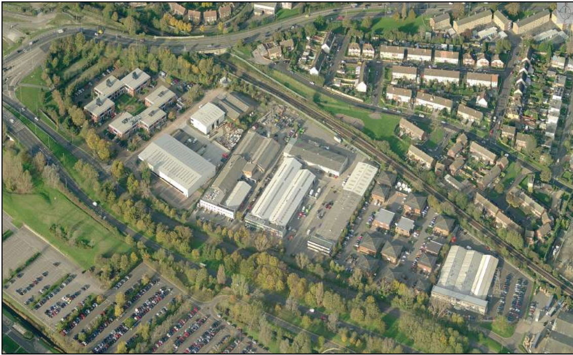
2. Oblique view from the south of sub-area A Western Road
