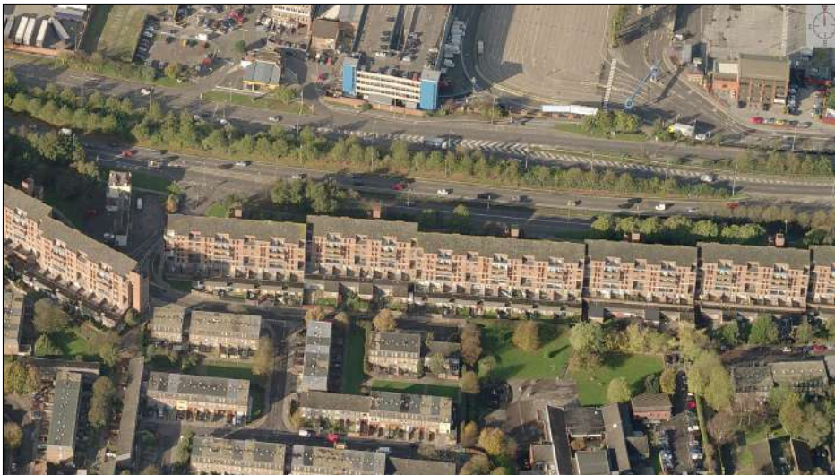
Central element of Estella Road Flats
