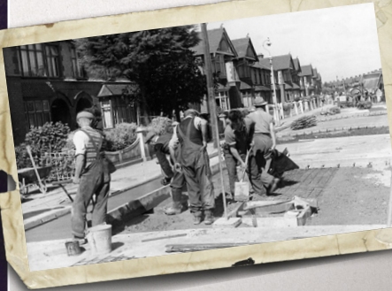
Work under way on the Highbury estate
