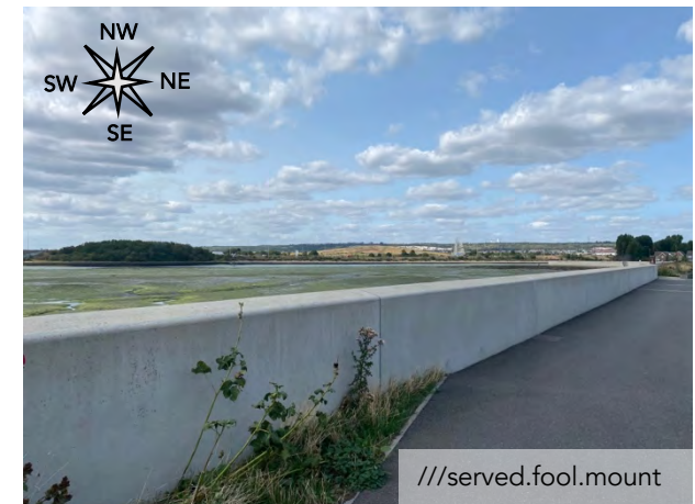
Photo 1f View over sea wall
