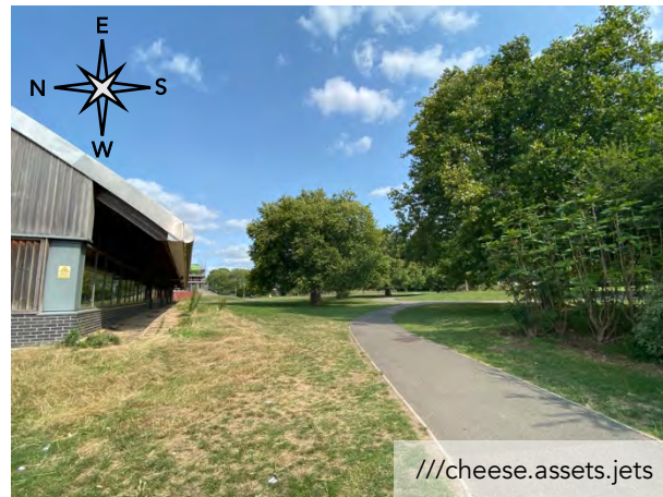
Photo 4c Back of Mountbatten centre and park
