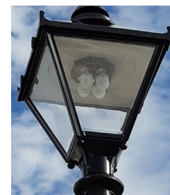
1200 LED lantern conversion, Heritage area, Phase 2
