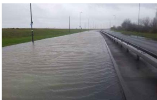
Figure 3-1 Overtopping along Eastern Road frontage, January 2015 (LFRMS)
