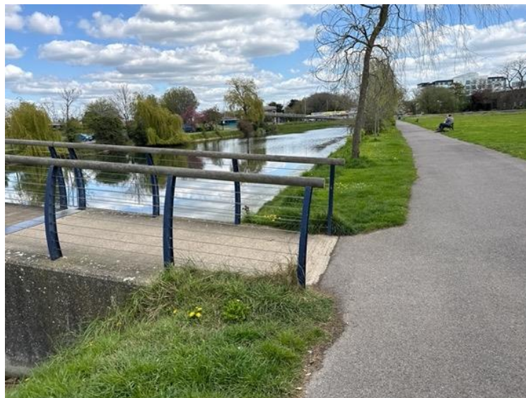
Photograph 2 : Bridge Across Waterbody
