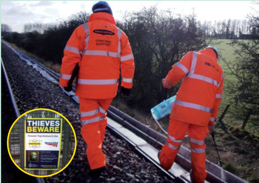
**Pictured:** SmartWater is applied to trackside cable
