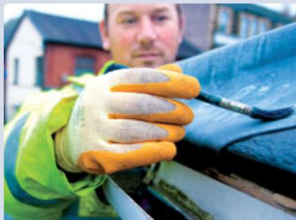
**Pictured:** SmartWater is applied to lead roofing on Pontypool Indoor Market
