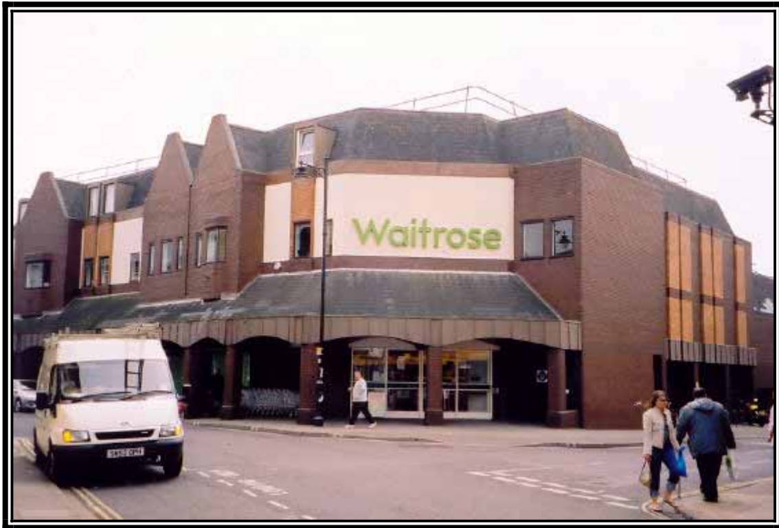
Photo 21: Waitrose, Southsea Town Centre
