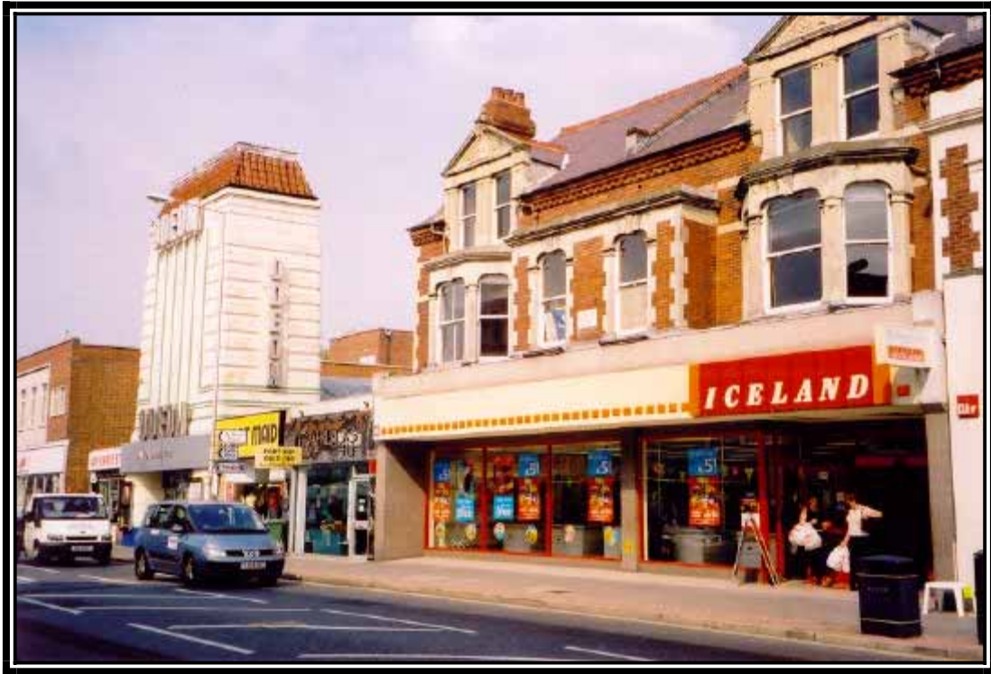
Photo 17: Iceland, North End/London Road Suburban Centre
