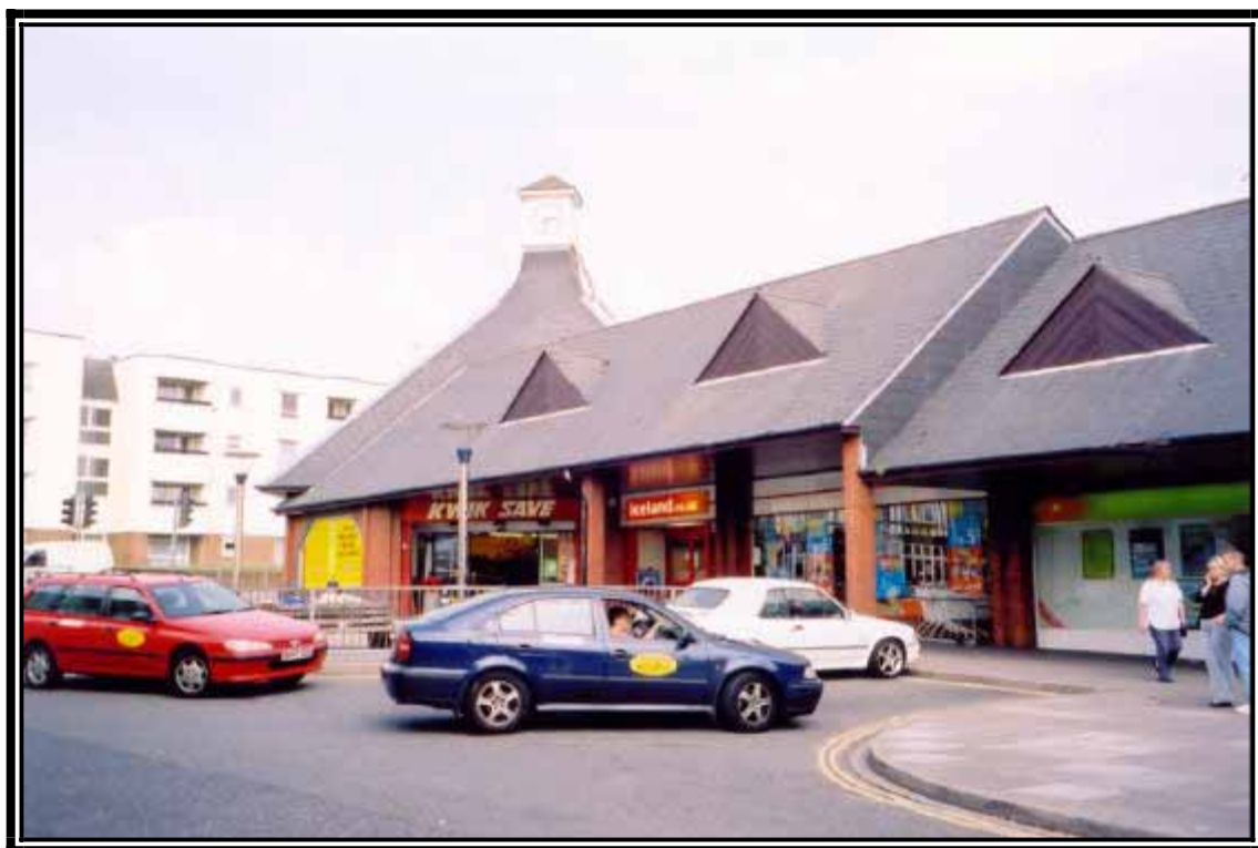
Photo 12: Kwik Save, Cosham Suburban Centre
