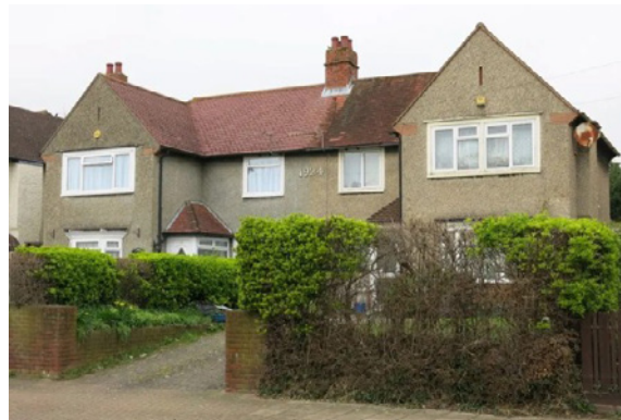
Houses on Medina Road, Wymering, dated 1924. Available from: https://municipaldreams.wordpress.com/2020/04/21/council-housing-in-portsmouth-part-i
