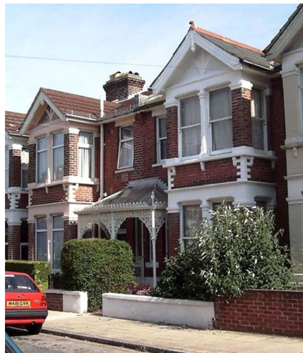
Double bay properties with right hand house retaining slate roof & sash windows
